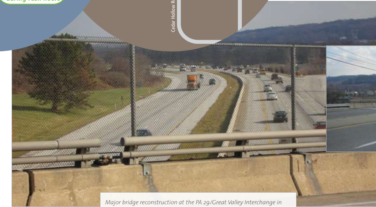
Major bridge reconstruction at the PA 29/Great Valley Interchange in 2008 and beyond will include replacement of the PA 29/Morehall Road overpass.
