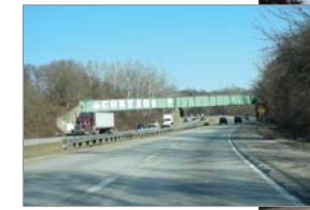
The Cedar Hollow Road overpass (above) will be replaced beginning in 2008 with a new bridge that will be constructed on a new alignment south of the existing span. An abandoned railroad overpass (inset) will be raised to increase the vertical clearance for vehicles on US 202.
